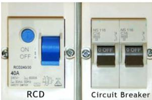
An RCD looks like a circuit breaker but also has a test button. The [attached photograph](#) shows two circuit breakers compared with an RCD (**note the test button**).
